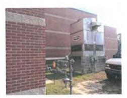
The cooling tower is an EVAPCO induced draft cooling tower, model USS 19-76. The assumed capacity is 125 tons to match the single chiller. The tower pumps are constant speed, base mounted, end suction pumps and the tower fans are constant speed.
